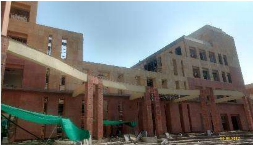
Food Court, Restaurant and Accommodation
